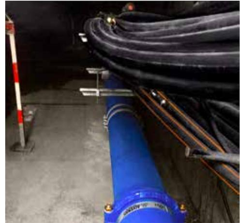
*No welding possible due to gas and power lines in the tunnel*
